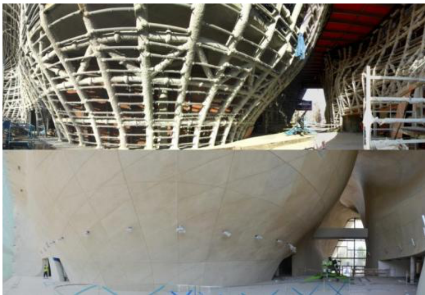
Fig. 3: The steel structure of the wall and the final visual, result of the discrete surface
